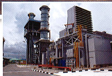
GAS TURBINE/ HEAT RECOVERY STEAM GENERATOR
